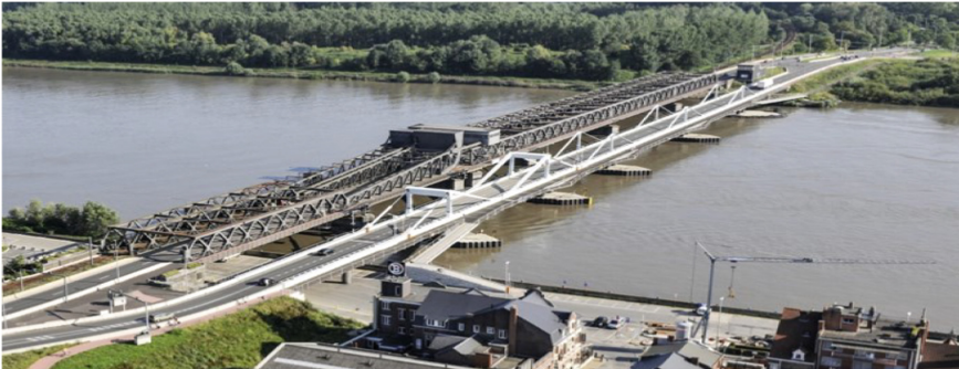
Fig. 1. Aerial view of the bridge, showing (from left to right) the studied railway bridge, the old road bridge and the newly constructed road bridge.
