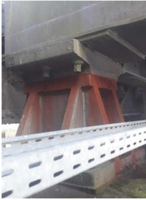
(a) Simply supported bridge bearing at transverse girder end
