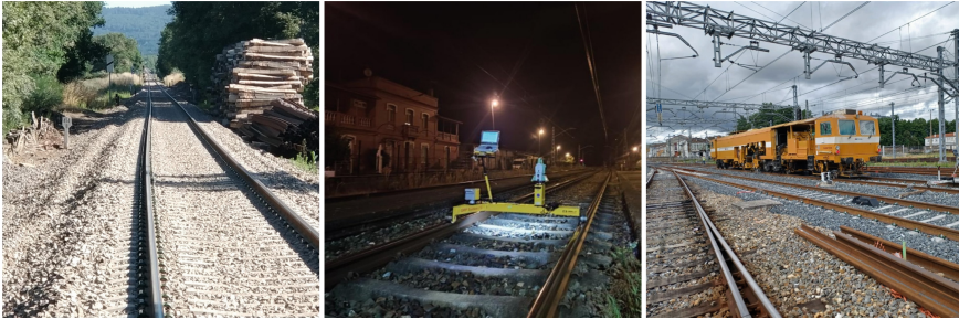
Fig. 1. Railway deviation, track surveying machine and tamping and lining machine.
